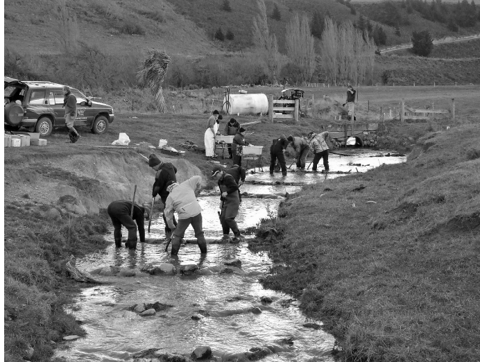
Hacketts Creek: Placing the Scotty Boxes in the Weirs
