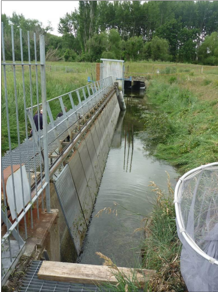
Figure 2. The dewatered forebay and screen, looking upstream toward the bridge and the control gate (left), and the downstream side of the screen while water was shut off. (right). Both photos were taken on 7 December 2010. Left photo by Sjaan Bowie, right photo by Nicholas Dunn.
